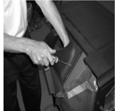
FIG. 14 Remove Flue Collar
