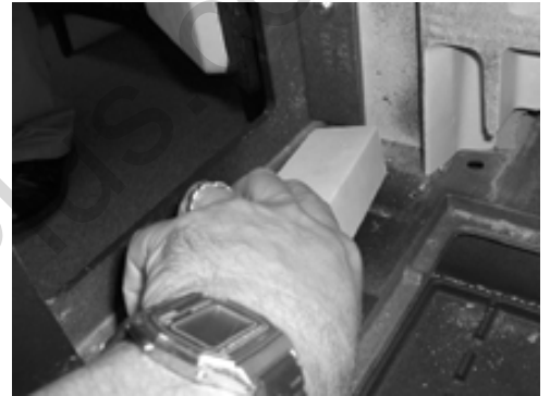
FIG. 6 Remove Lower Load Door Refractory
