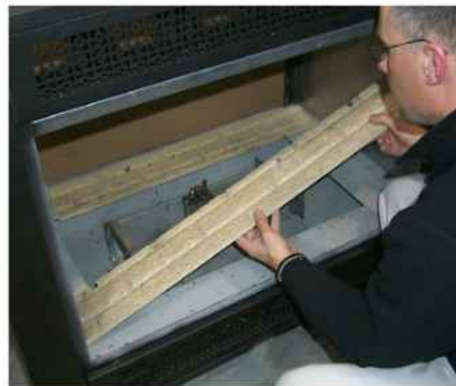
Remove the 2 Long Base Brick Panels
