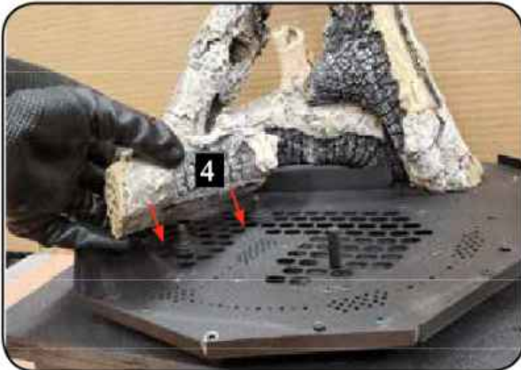
Log 4 - install onto pins on burner
