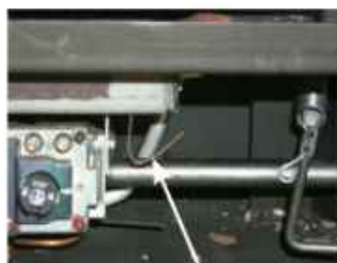
Adjustment wire: Push to close or pull to open aeration cap.
