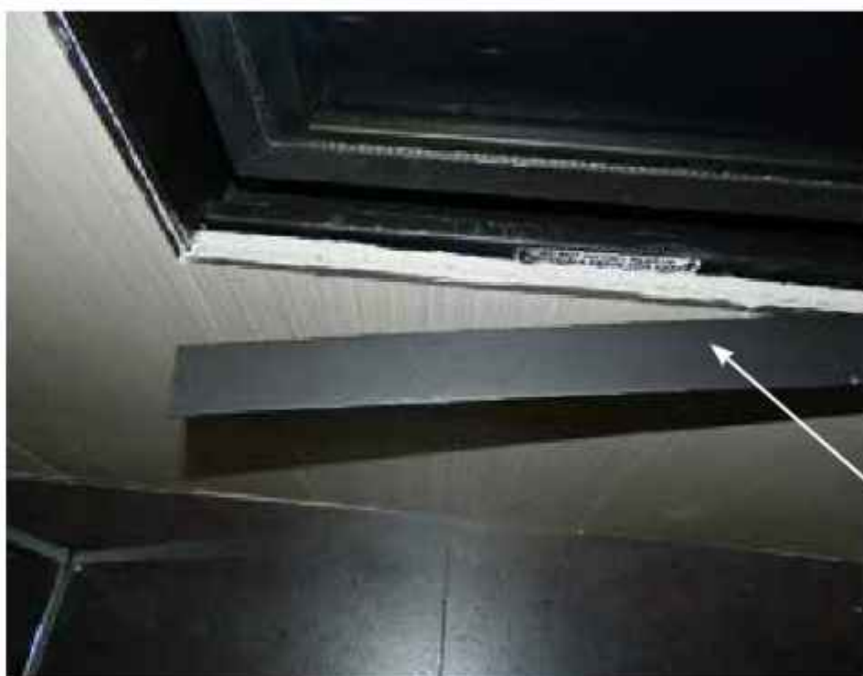
Figure 101: Top View - Sliding trim into place
