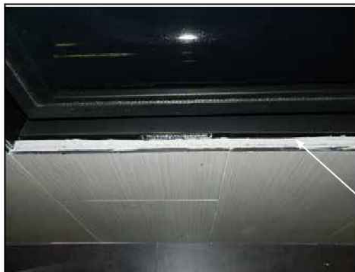
Figure 100: Top View - exposed non combustible materials
