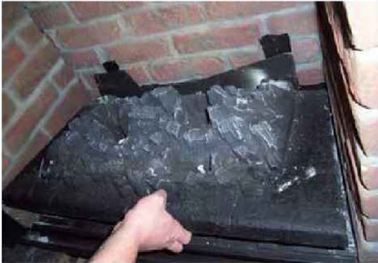
Figure 79: Burner Removal
