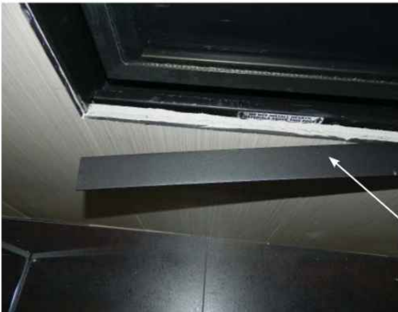
Figure 101: Top View - Sliding trim into place
