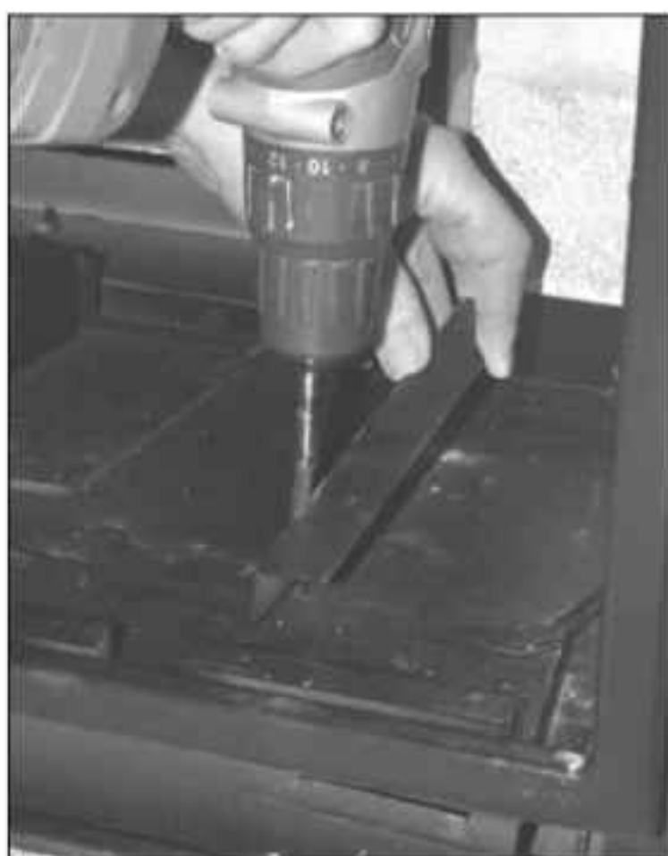
Figure 56: Removing the Right Burner Support.
