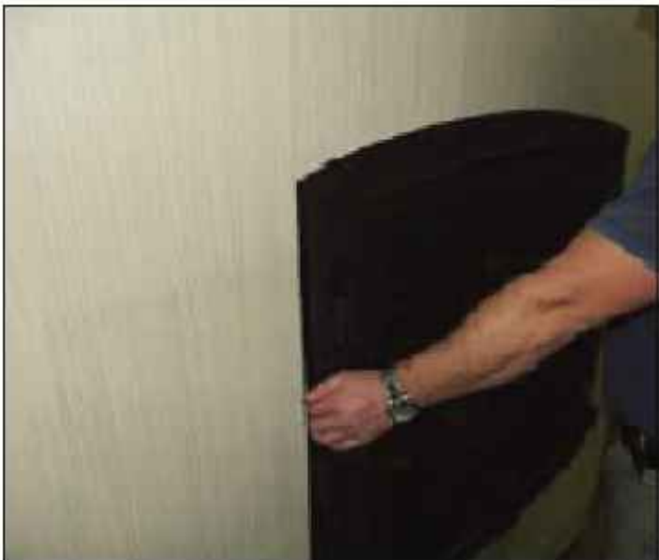
Safety screen installed
