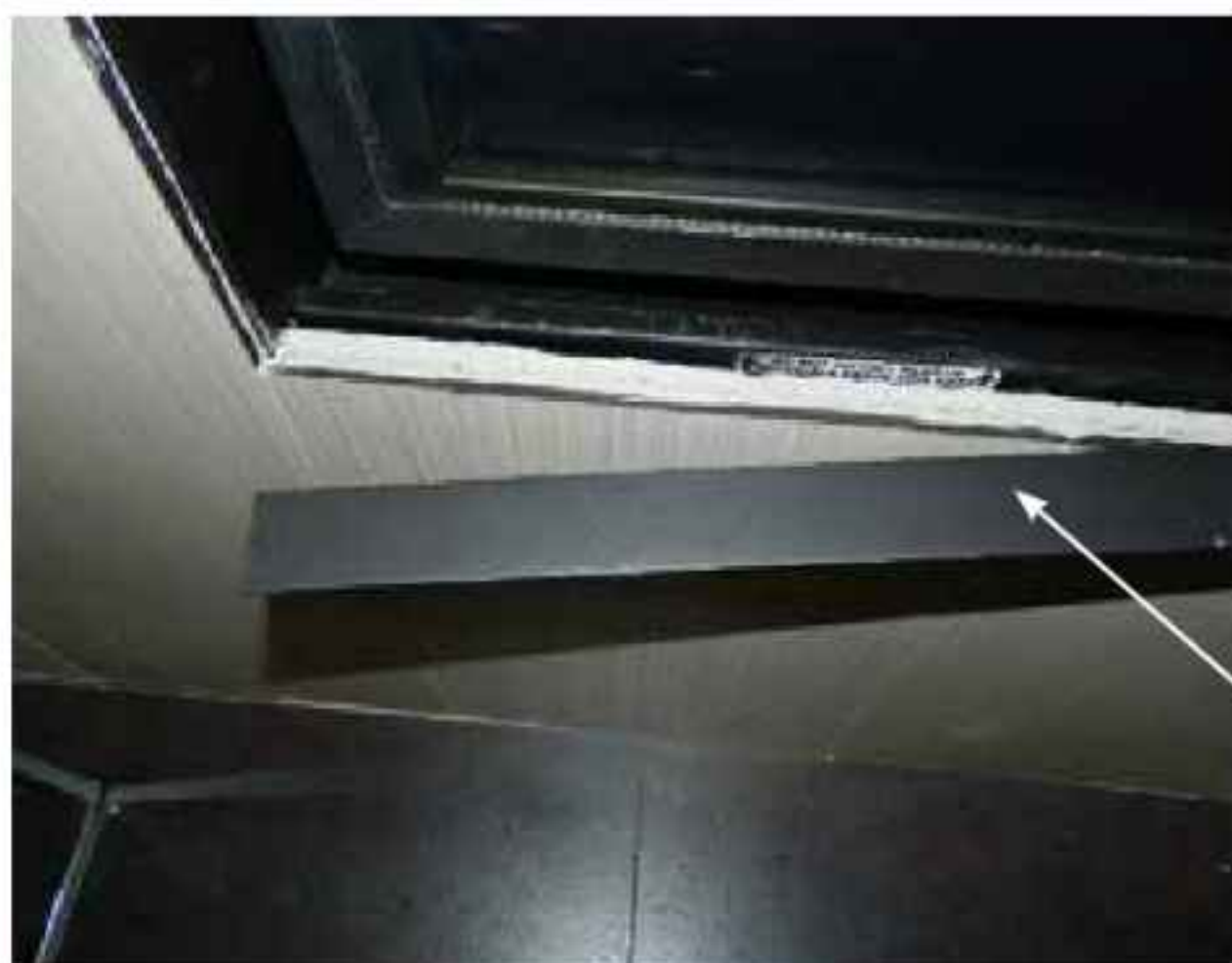
Figure 101: Top View - Sliding trim into place
