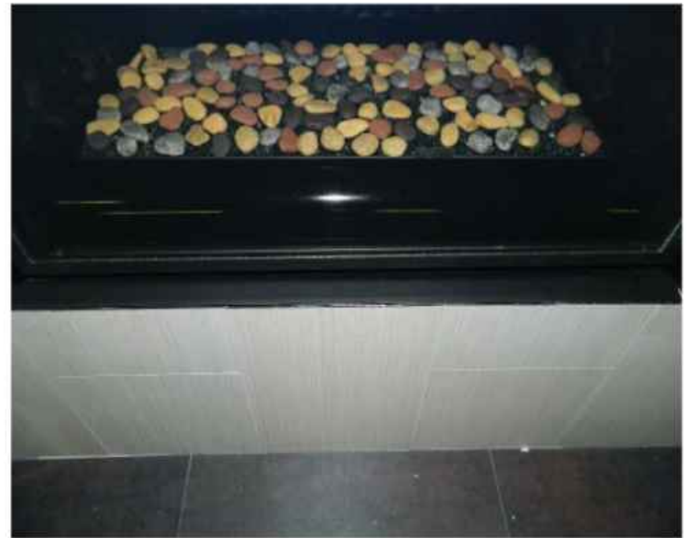
Figure 102: Completed Trim install
