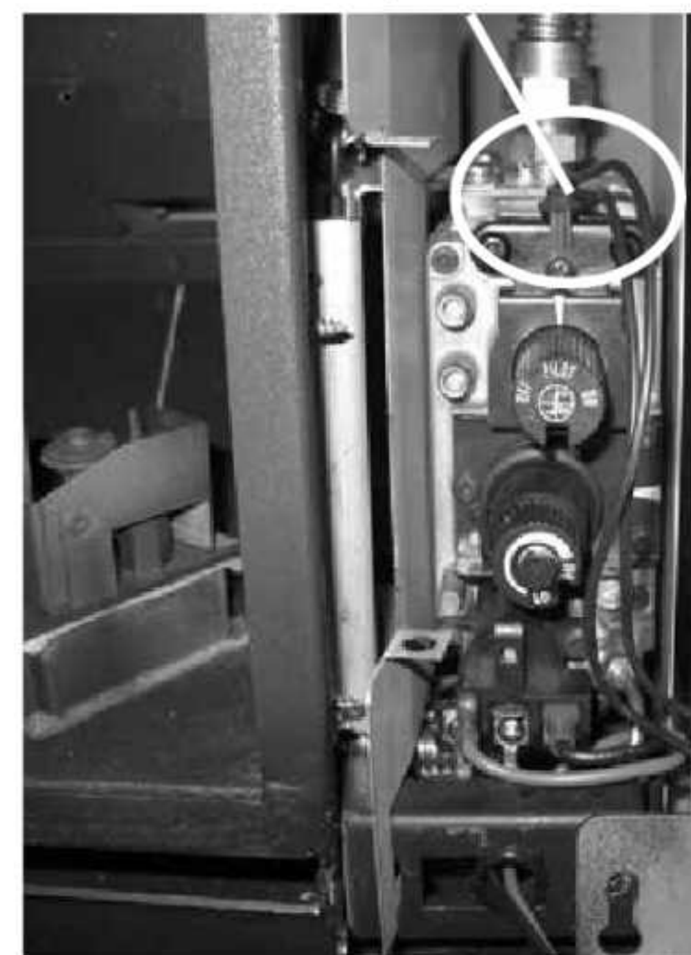
DC Sparker Wires
