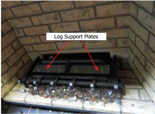
Diagram 6—Log support plates installed
