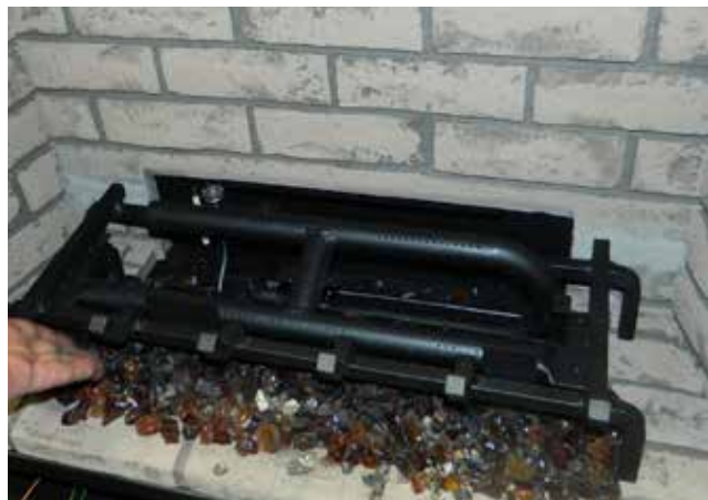
Diagram 4—Install Vermiculite + Lava
