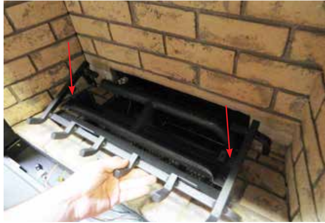
Diagram 2—Log Grate Install
