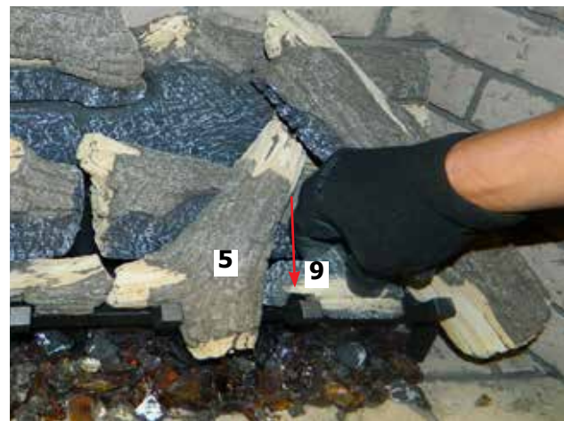
Diagram 15—Install Log 9
