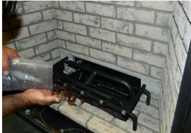
Diagram 3—Install Glass
