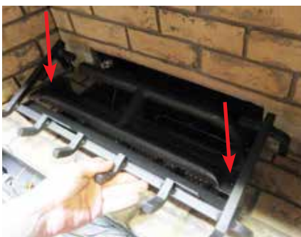
Diagram 1: Remove the left and right screws.
