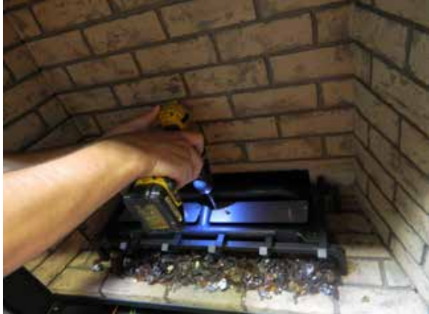
Diagram 5—Install Log support plates
