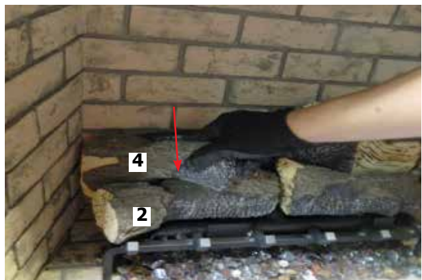
Diagram 10—Install Log 4
