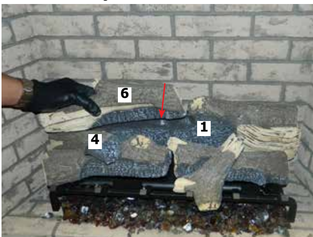
Diagram 12—Install Log 6
