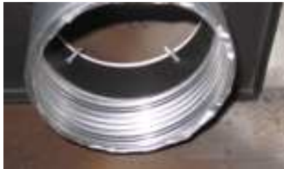
Secure top plate to firebox w/4 screws.
