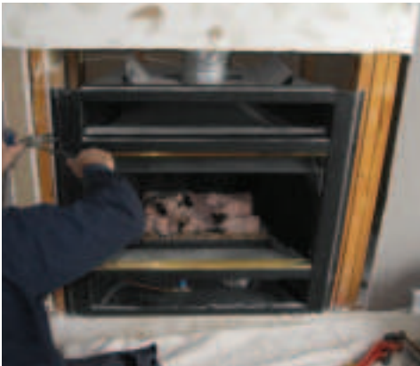
Remove unit from framing
