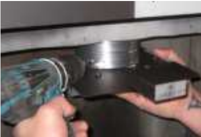
Secure vent slide plate to flex pipe with 4 screws
