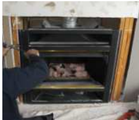
Remove unit from framing
