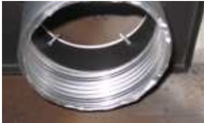
Secure top plate to firebox w/4 screws.
