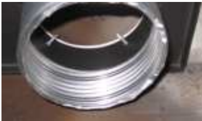
Secure top plate to firebox w/4 screws.
