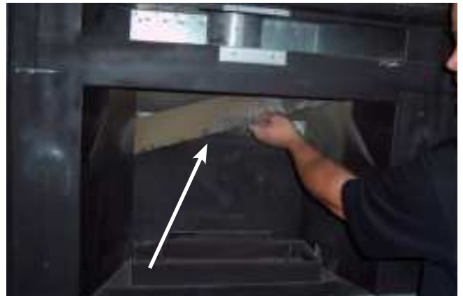
Remove rear baffle.
