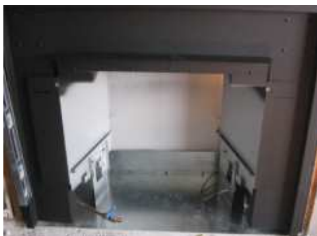
Outside firebox shown in position - refer to measurements (Step 22) before securing to surround.
