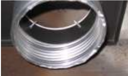
Secure top plate to firebox w/4 screws.
