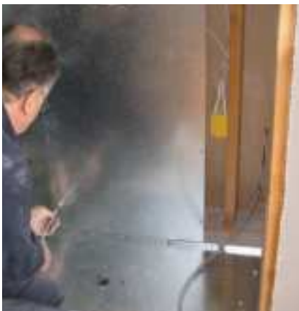
Fasten ZC box sections with provided screws.
