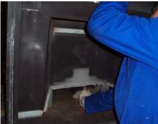
Flatten louver brackets
