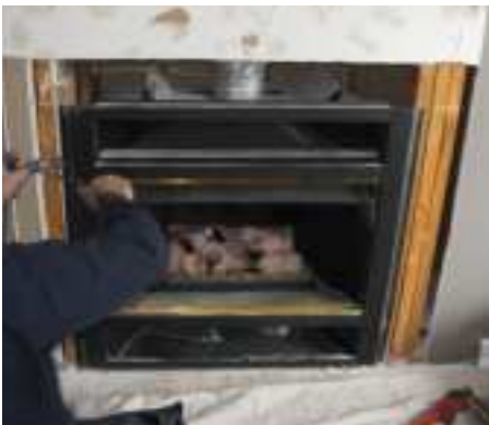
Remove unit from framing
