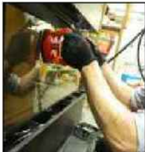
Handle glass with supplied vacuum clamps
