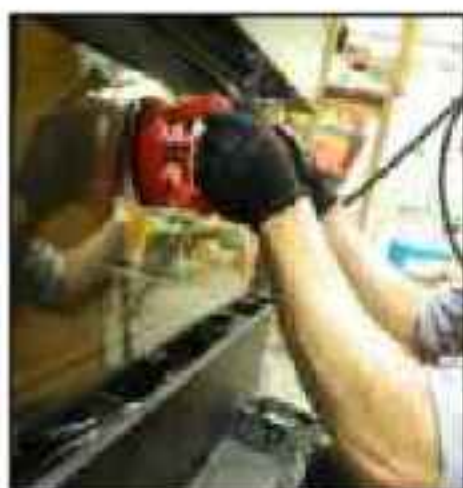
Handle glass with supplied vacuum clamps
