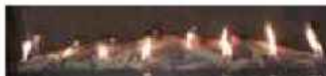
Correct main burner flame pattern
