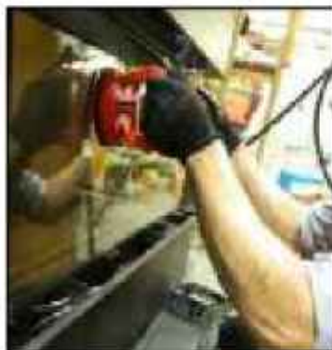
Handle glass with supplied vacuum clamps
