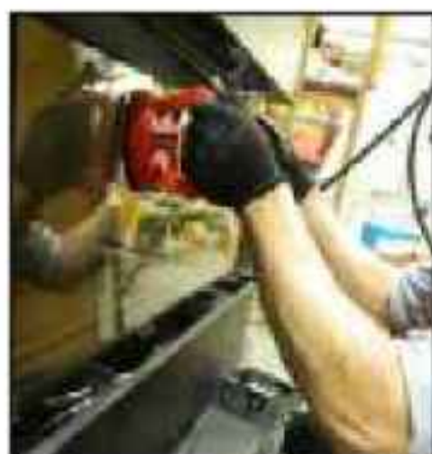
Handle glass with supplied vacuum clamps
