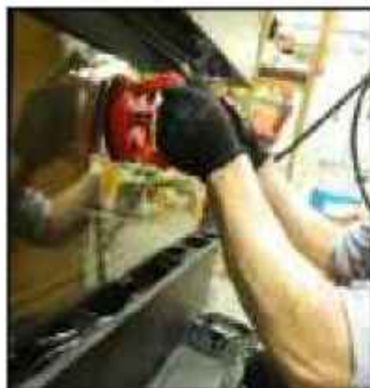
Handle glass with supplied vacuum clamps
