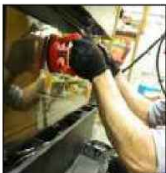
Handle glass with supplied vacuum clamps
