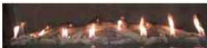
Correct main burner flame pattern
