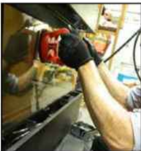
Handle glass with supplied vacuum clamps.
