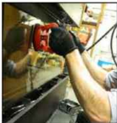
Handle glass with supplied vacuum clamps
