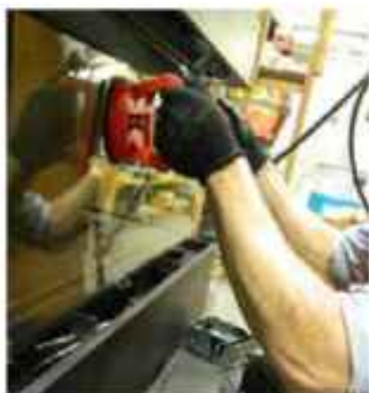
Handle glass with supplied vacuum clamps
