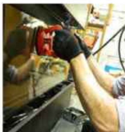
Handle glass with supplied vacuum clamps
