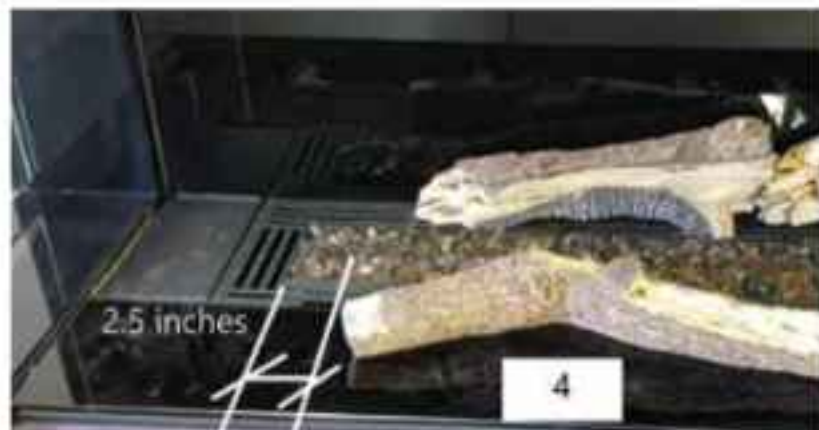
Log 4 to edge of burner
