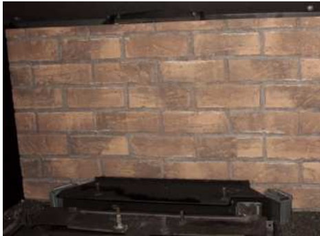
Back Panel Installed
