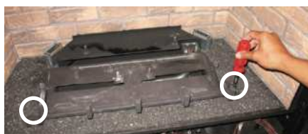
Diagram 1: Remove the left and right screws.
