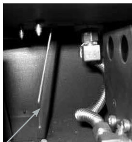
Air shutter rod - located to the left of the valve assembly.
