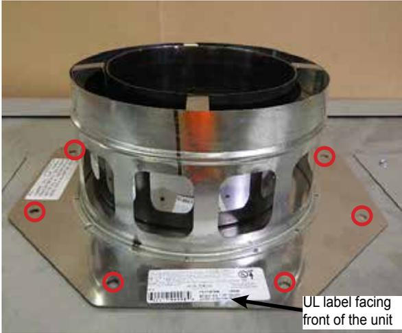
**NOTE:** While attaching the metal fab/anchor plate/starter collar, the UL label should be up and facing the front of the unit.
