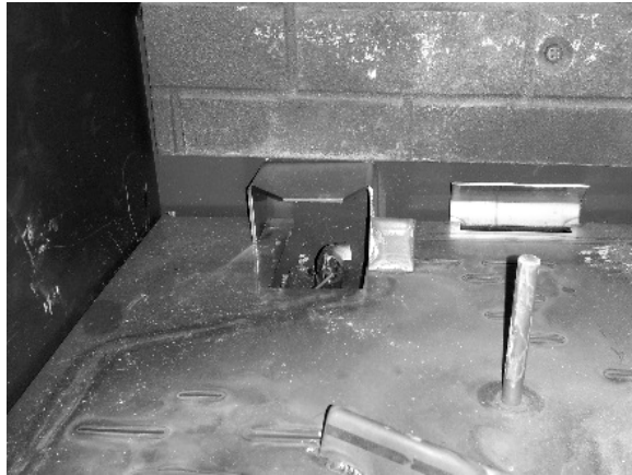
Figure 6 – Pilot, Shield, and Burner Position
