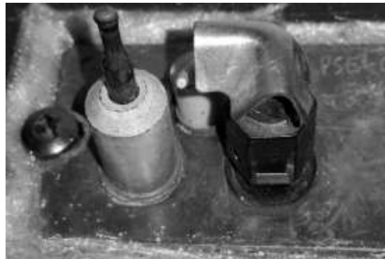
Figure 4 – Correct Pilot Hood Orientation
