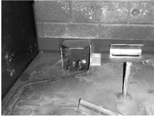
Figure 12 – Pilot, Shield, and Burner Position
