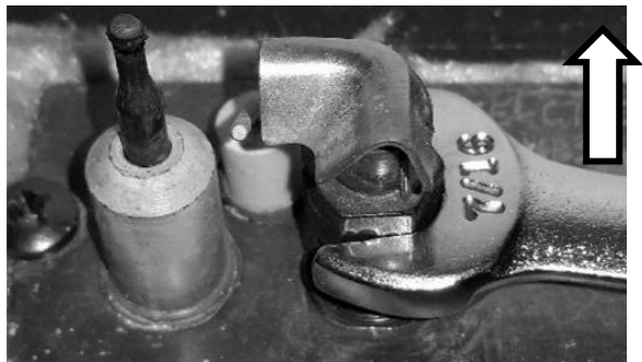
Figure 8 – Loosening Pilot Tower
