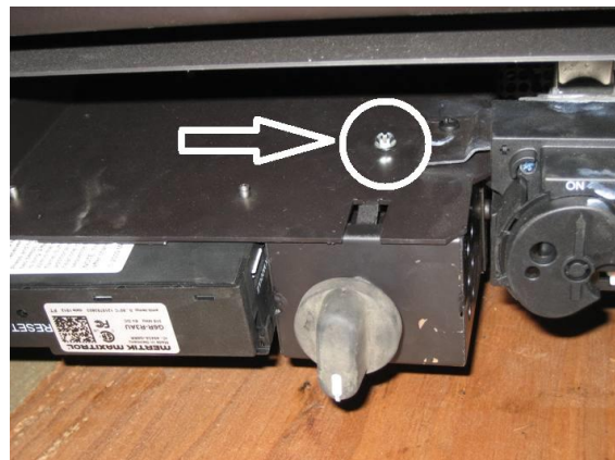
Photo #9 – Tilt Valve Tray Down and Install Screw
