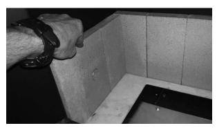
18. Install the firebox floor plate (if unit has been burned use a new floor plate gasket) and install floor bricks.
