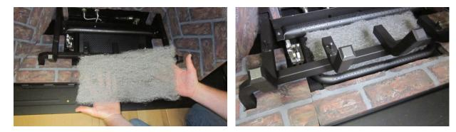
3. Place 1 bag of ember chunks over the stainless steel. The chunks should not cover the burner or any of its ports.
