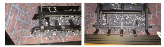
5. Tear small chunks of rock wool and place them over the burner as shown below. They should form a loose layer over the burner that allows for air to pass through. <u>USE THE ENTIRE BAG OF EMBERS</u>.
